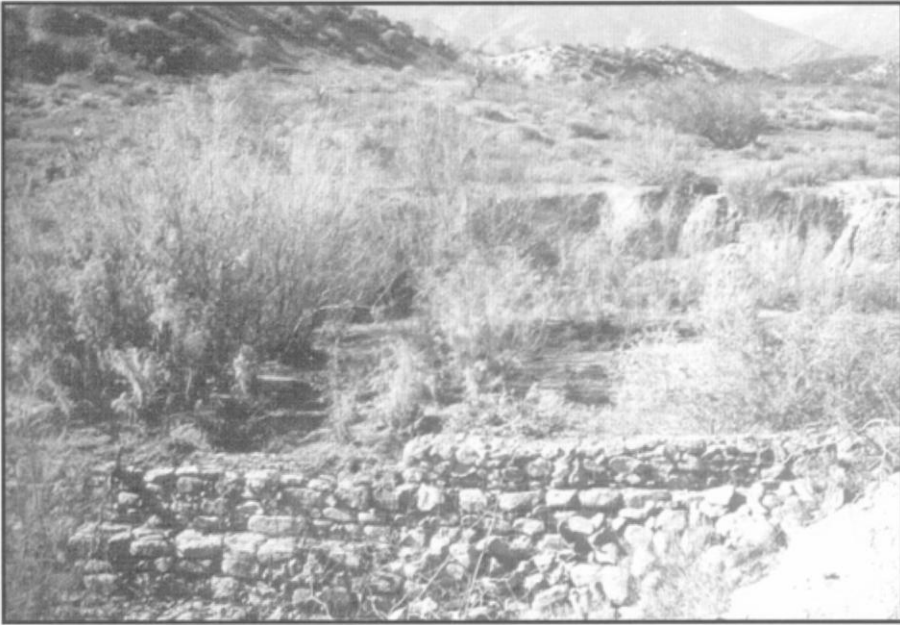
Same Check Dam in 1944. The growth and increase are from protection and planting. Note surface area still mostly bare, suggesting the mixed results of CCC work. Photo by George D. Hardaway. Courtesy of the Tonto National Forest.
